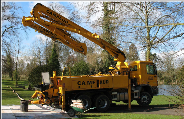
An off the back job with 200m of pipeline
