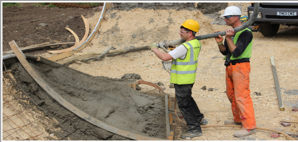
Concrete spraying using M20 pump
